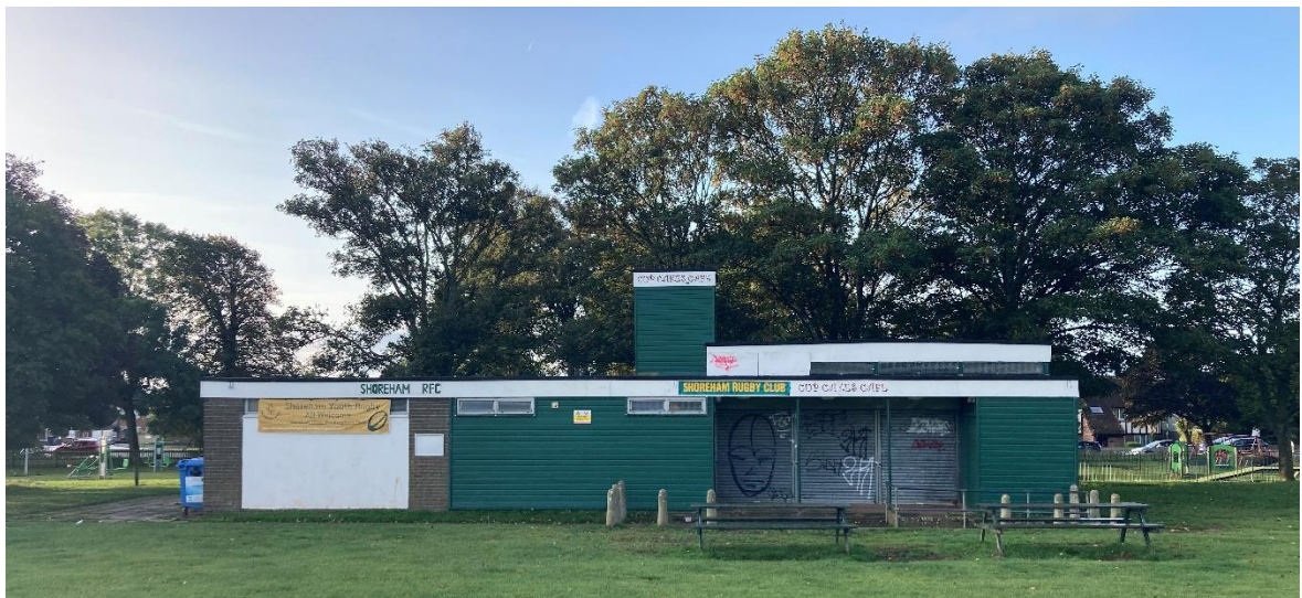
Figure 3- Existing Building (North Elevation)
